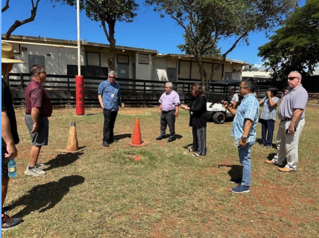
Talking over a sinkhole about the troubled field
