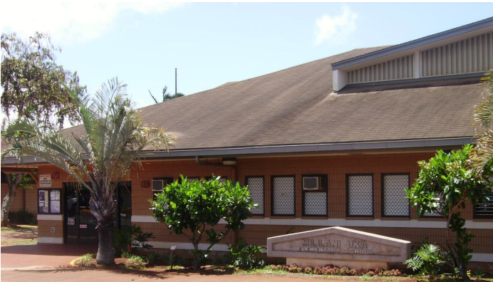
Campus upgrades underway at Mililani Uka Elementary (above)
