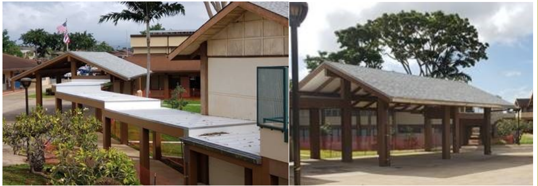
Kalei'opu'u Elementary School's completed covered walkway.
