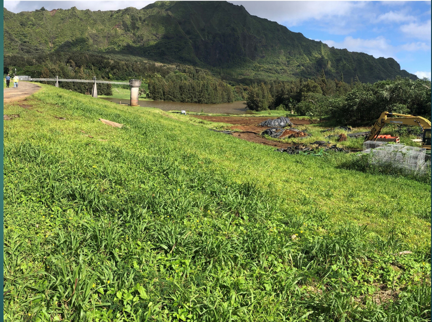
Nuuanu Dam No. 4, Oahu
