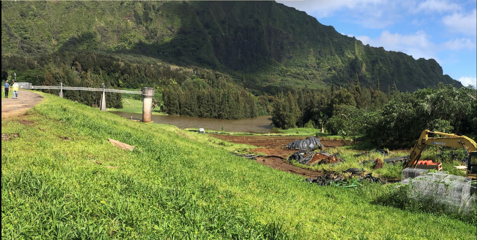
Nuuanu Dam No 4, Oahu (Improvements, Feb 2021)
