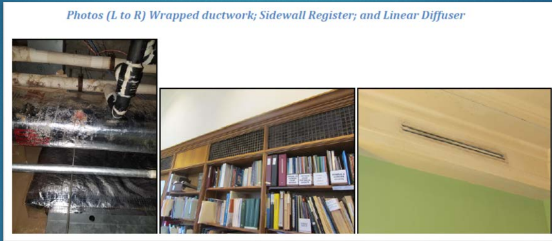
Wrapped duct work; Sidewall register; Linear diffuser
