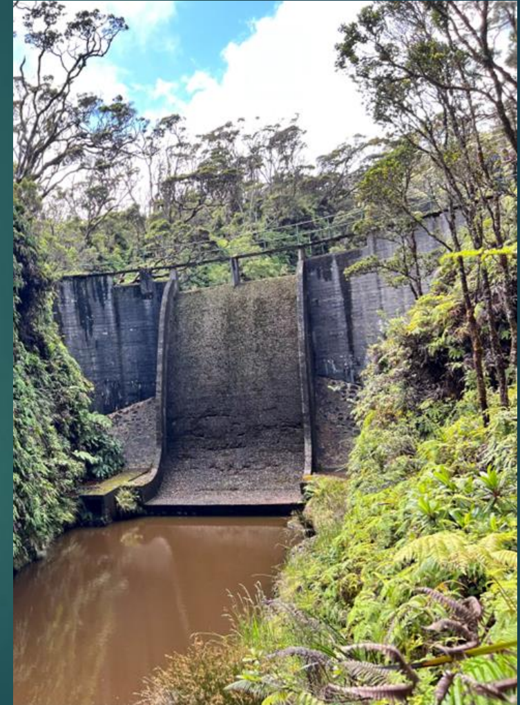
Waikamoi Dam No. 2 Spillway, Maui (MA-046)
